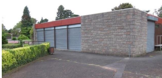
Figure 12 The old pavilion
