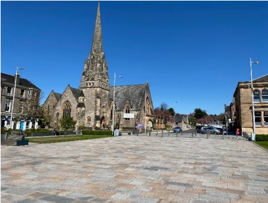
Figure 4 Restoration work at Colquhoun Square
